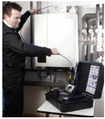
The 360° pan and 180° tiltable color camera head easily negotiates 90° bends.
